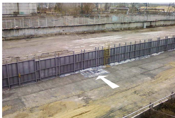
Fig. 8. An example of shielding with powerful gamma-radiation lead on sites [1] that were predicted due to gamma- and spectrometric gamma-logging results
