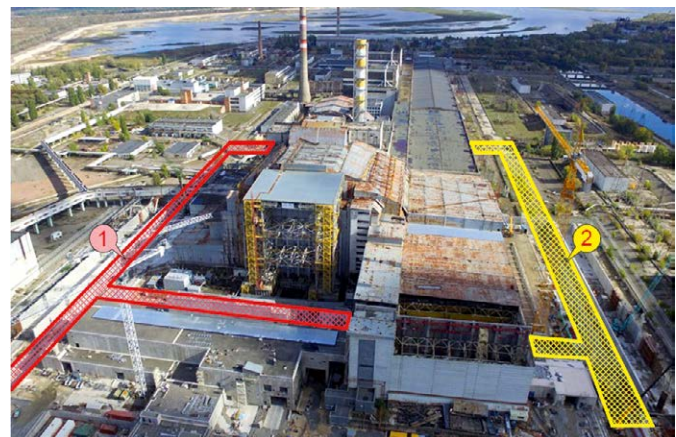
Fig. 1. General view of the Shelter object: 1 – the northern foundation zone; 2 – the southern foundation zone
